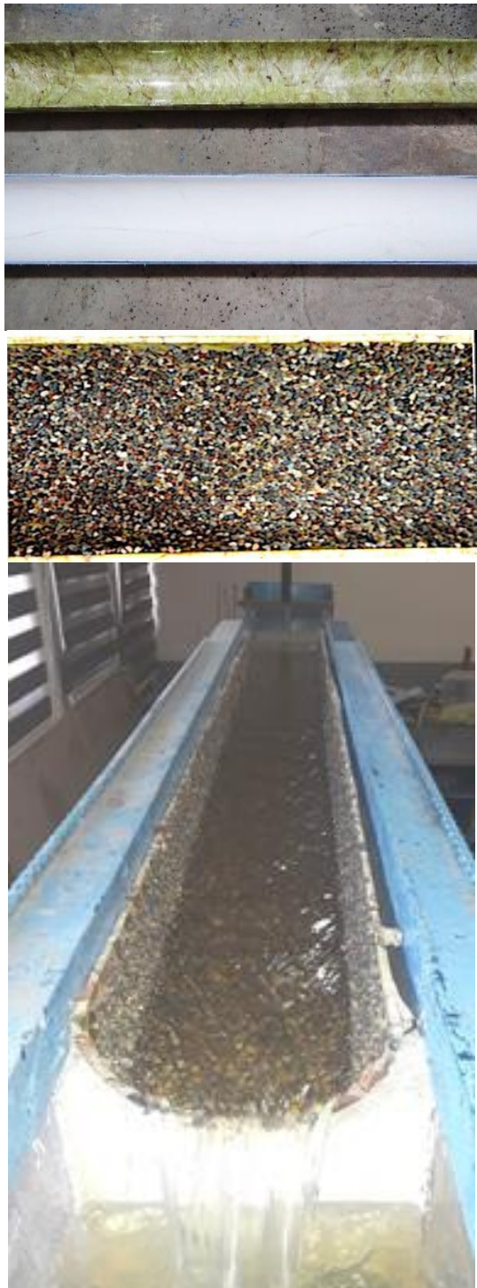
Fig. 4 Stages of installing the roughness layer
