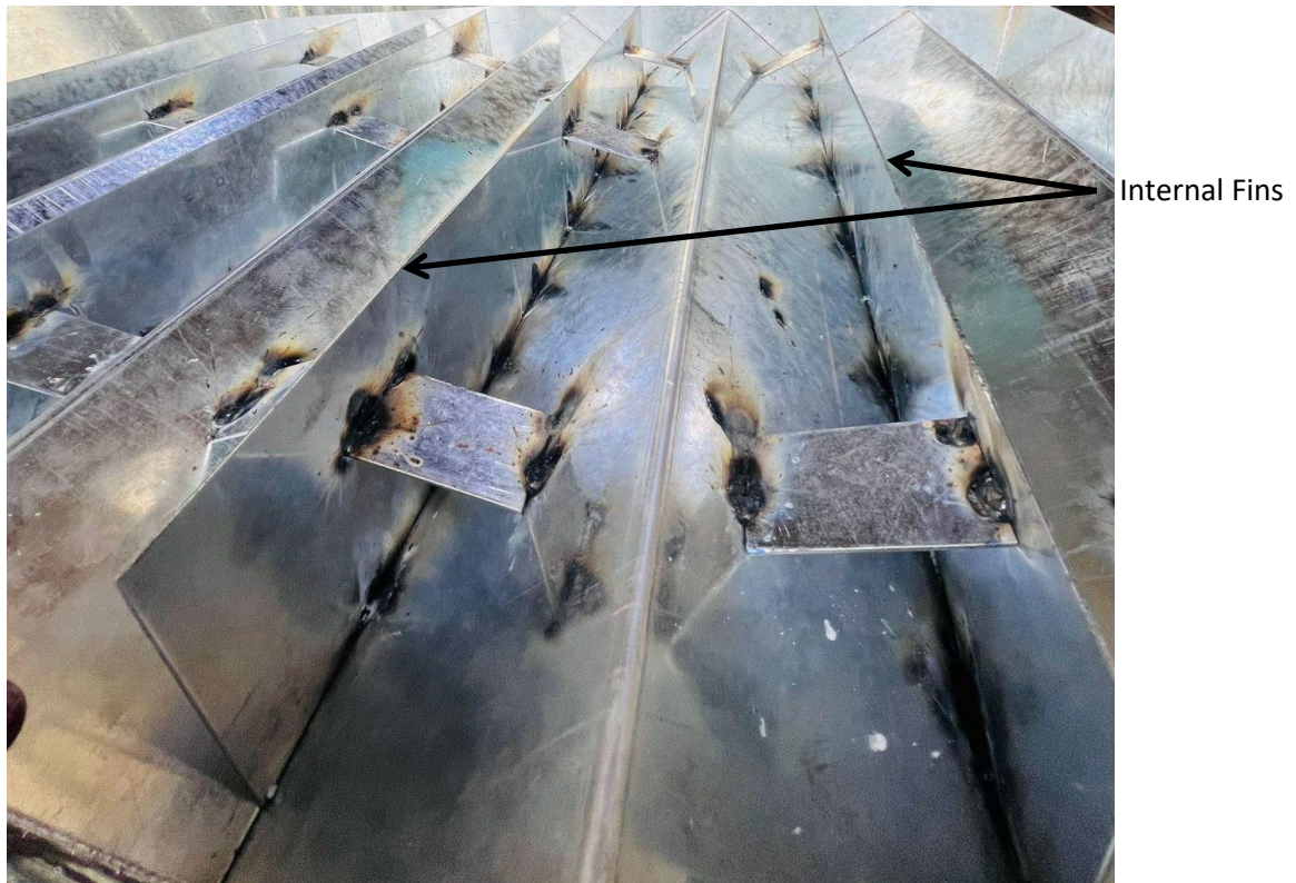
Fig. 2 Fins Inside the Storage Tank.
