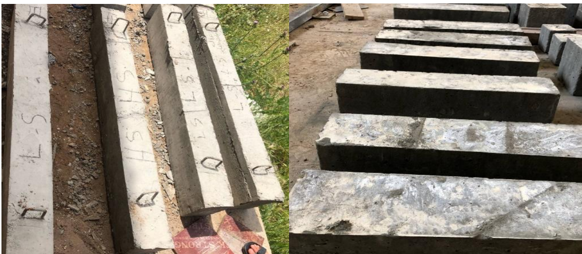
Fig. 9 Beams After Opening the Molds.
