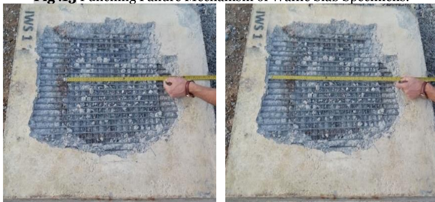
Fig.14 Punching Shear Failure Angle Measurements of Control Specimen IWS1.
